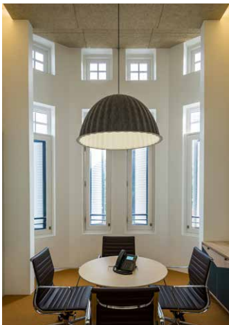
Double volume space reinstated to expose fanlights
